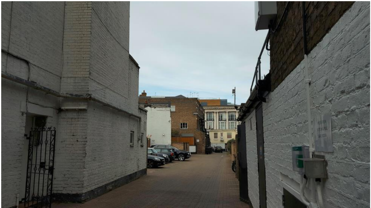
View of site in Moscow Road (top) and view along Queen's Mews from Moscow Road (bottom).
