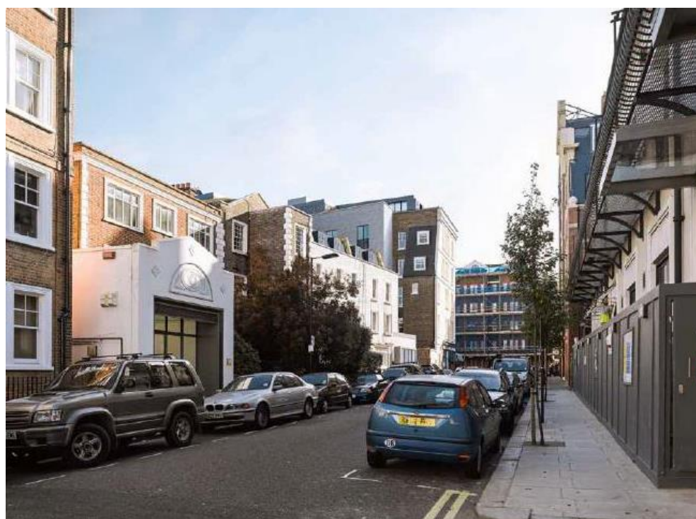
Photomontage of proposed Moscow Road elevation (top) and photomontage of proposed rear elevation (bottom).
